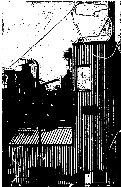
Shown above is the first commercial scale MIVAC plant, a microwave/vacuum crop drying system that evolved from space simulation technology. The pilot MIVAC, located in Guntersville, Alabama, is operated by Continental Grain Company; the spinoff system was developed by McDonnell Douglas Corporation.
