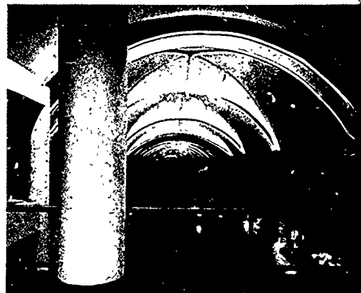
The trend-setting Mall At 163rd Street, Miami, Florida, was the first shopping center to be completely enclosed by a permanent Fiberglas fabric roof. In this nighttime view, the roofing material reflects and diffuses interior lighting to provide soft, glareless illumination.
